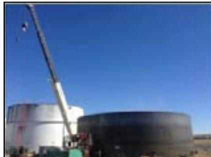
*Construction is underway on the additional 1.5 million gallon ethanol storage tank.*
